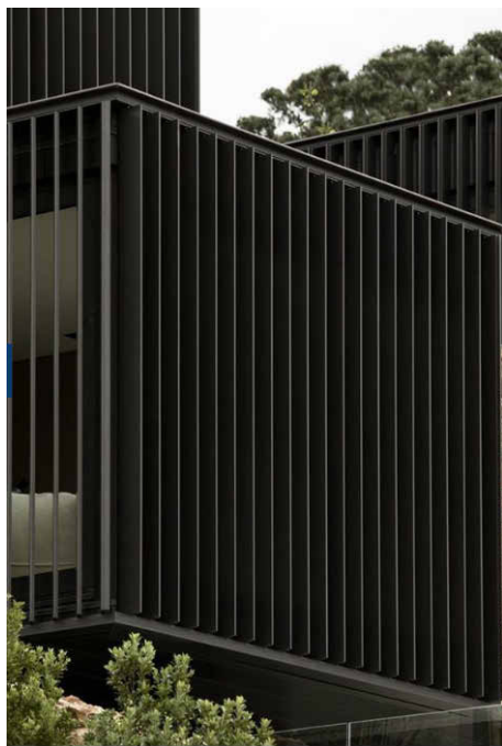
02 - CHARCOAL VERTICAL LOUVRES CHARCOAL VERTICAL LOUVRES FOR SOLAR SHADING AND PRIVACY
