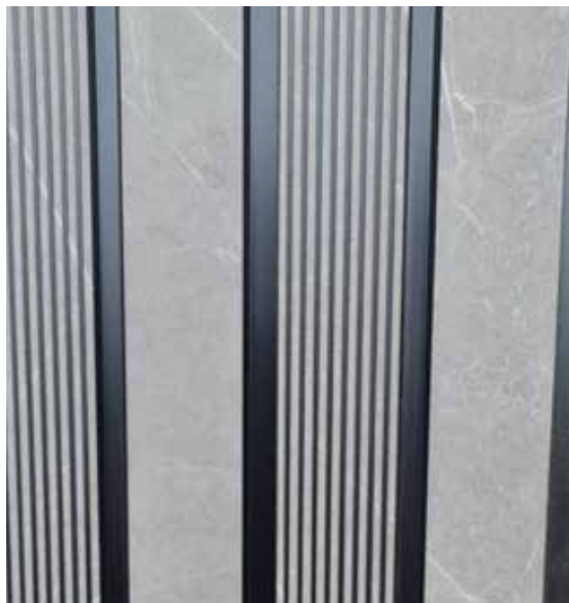
05 - CONCRETE "LOOK" VERTICAL LOUVRES GRC CLAD "CONCRETE LOOK" VERTICAL LOUVRES
