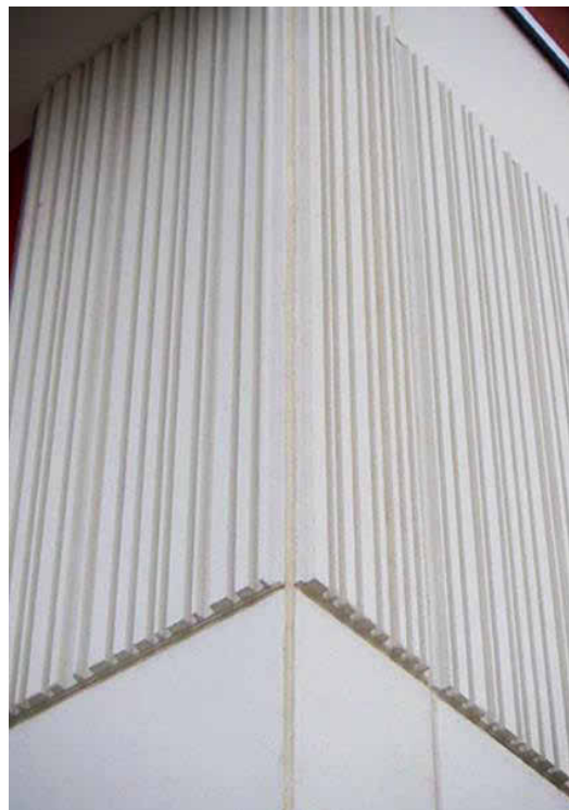
06 - CONCRETE TEXTURED FORMLINER CONCRETE TEXTURED FORMLINER TO FACADE FRAMES AND FEATURE WALLS.
